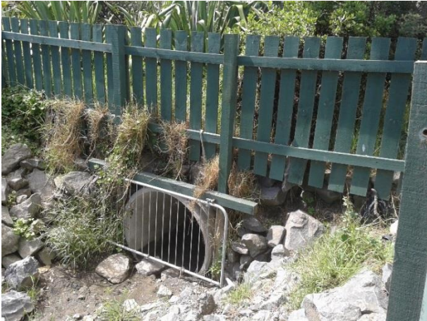
Figure 1 - Cynthia Pl stormwater outfall showing recent erosion repairs
