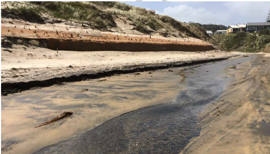
Figure 5 Photo of wall not long after initial construction complete (~2015)
