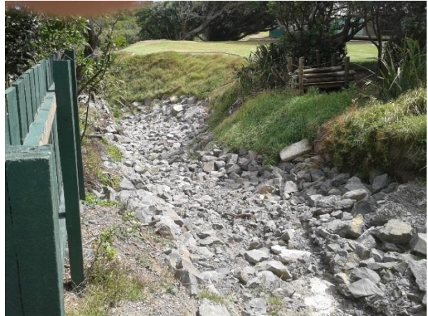
Figure 2 - Cynthia Pl (2) stormwater outfall showing recent erosion repairs
